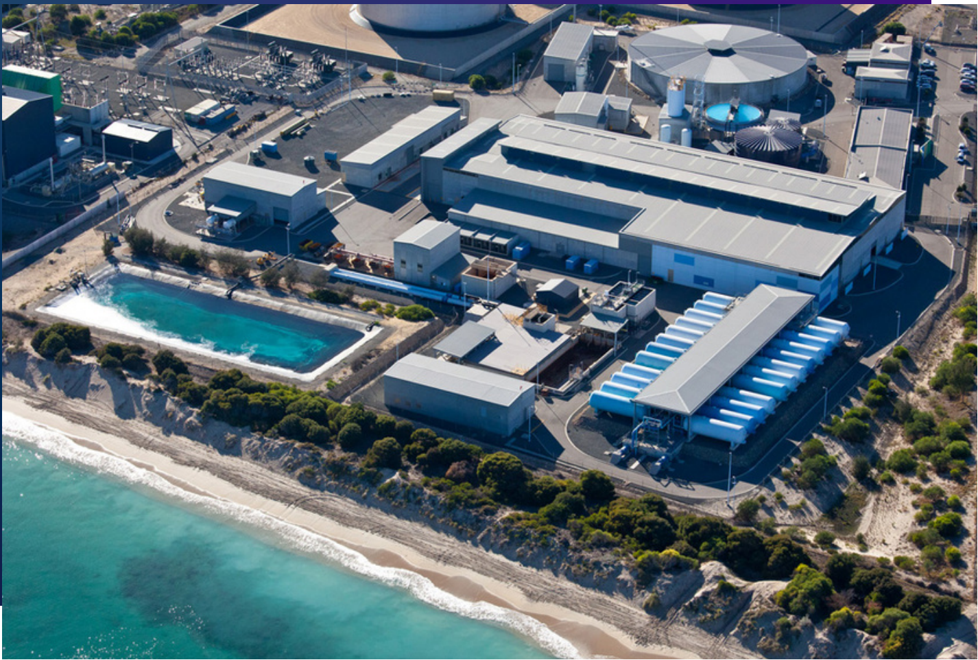
Perth reverse osmosis desalination plant
